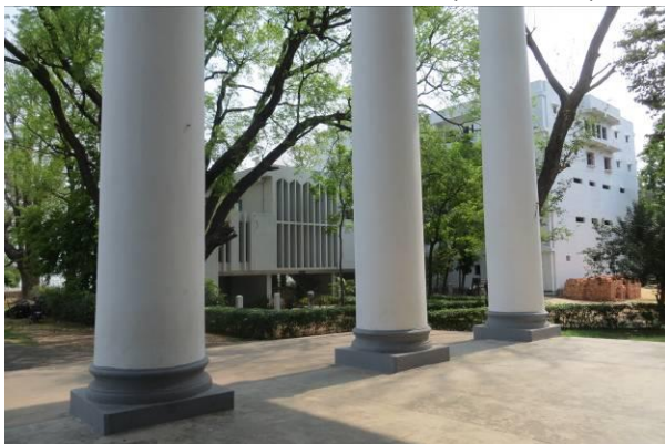
Looking to the Carey Library and the new build
